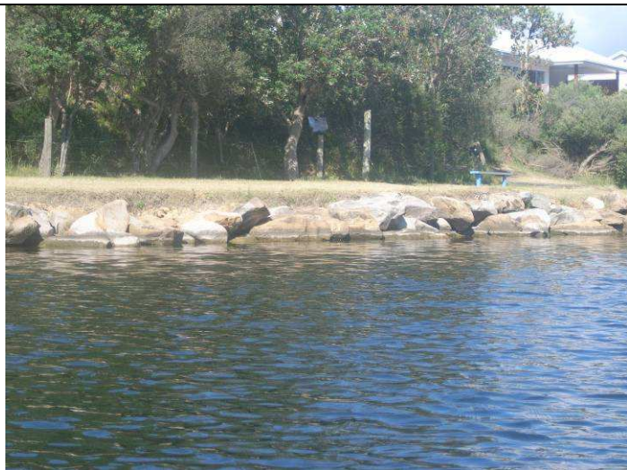
Photo 31: Bank protection works near the mouth of the lagoon
