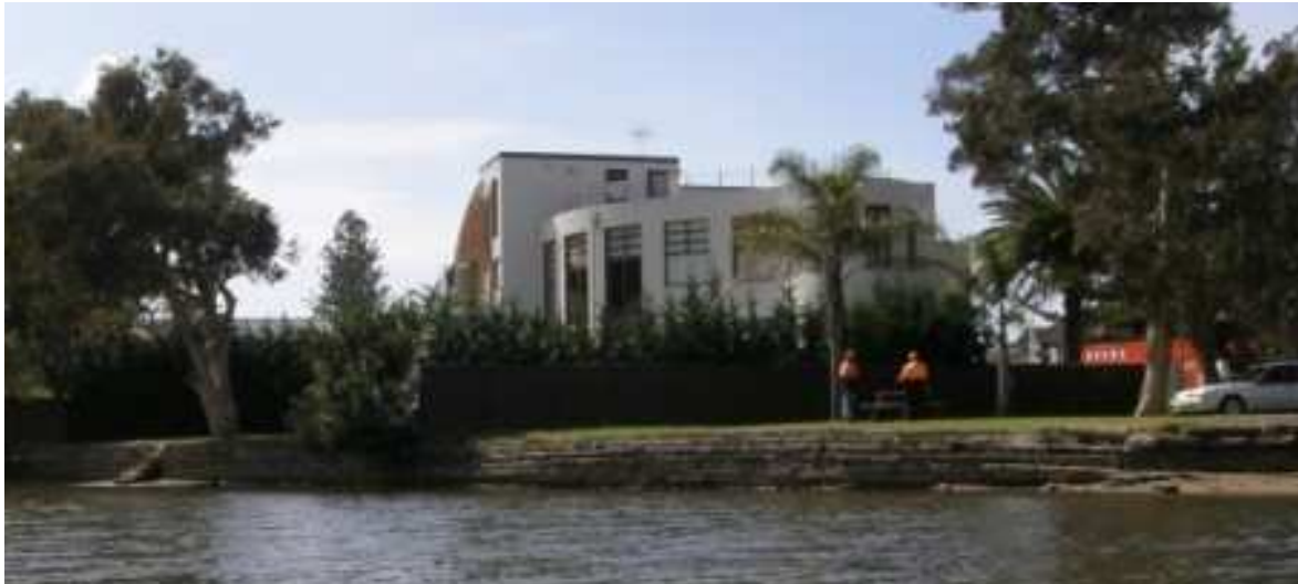
Figure 1.13 Example of seawalls on Terrigal Lagoon
