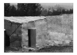
Figure 3 | A simple mushroom-growing house made from locally available materials, including bamboo.
