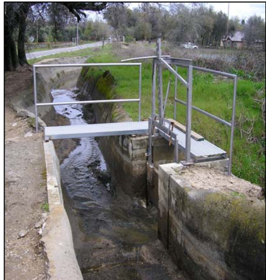
Boardman Canal at Hanson Spill dewatered and prepared for cleaning
