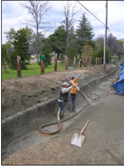
Baughman Canal lining
