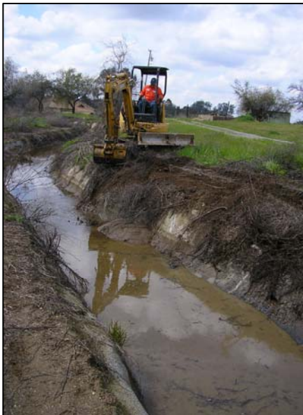
Debris removal from Baughman Canal
