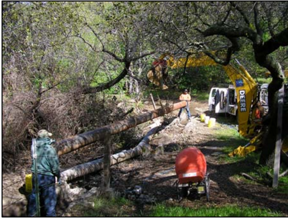
Barton Canal pipe replacement
