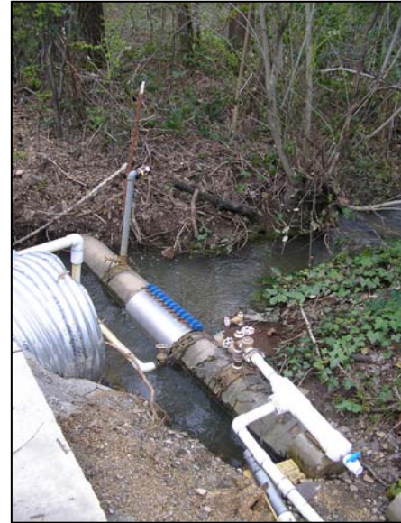
Pipe repair performed on PCWA canal
