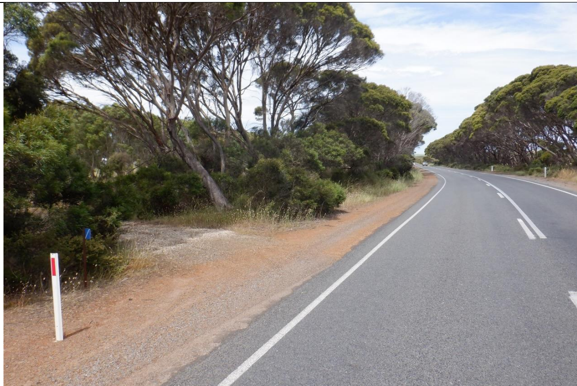
Photo 2621 facing south-west. Lat/Long: 35.7315 / 137.5672
