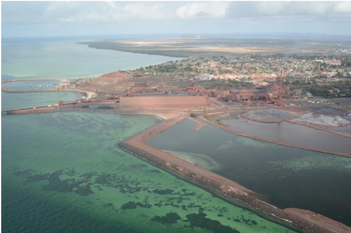
FIGURE 6.60 Looking south across the steelworks, port and city of Whyalla. Photo: Coast Protection Board, 2018.
