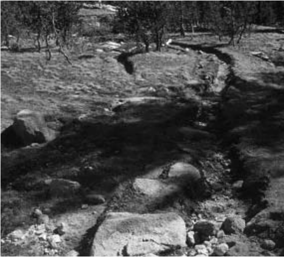
A trail in need of restoration and relocation. Note the multiple channels, eroded ground, and damage to the meadow.
