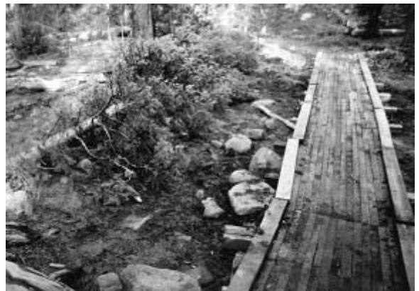
A boardwalk built to allow ground damaged by too many hooves and boots to recover.
