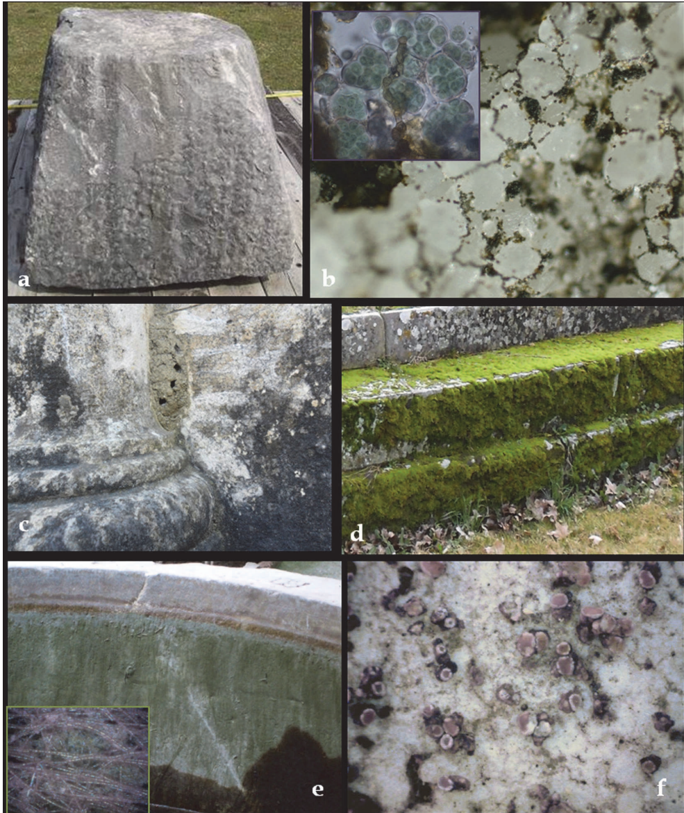
Fig. 7. Different patterns of biological growths found on monumental stones: (a) homogenous black crust with a detail (b) of intergranular development of threadlike microcolonies containing cyanobacteria and black fungi, Carrara Marble Museum, Italy; (c) heterogenous lichenic black crust with a wasp nest on a limestone tomb, Trespiano monumental cemetery; (d) bryophite extended carpets, Fiesole archeological site, Italy; (e) fibrous microbial mat with a filamentous diatom ( Melosira sp.) as a dominant species, Lindaraja Fountain from Alhambra complex, Granada (Spain); (f) micropits containing the apotheci of an endolithic lichen, Trespiano monumental cemetery
