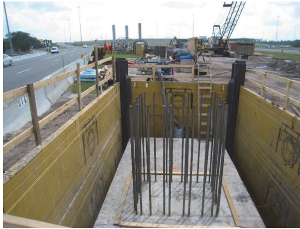
Figure 3. Bridge footing for monitoring in Orlando, Florida.
