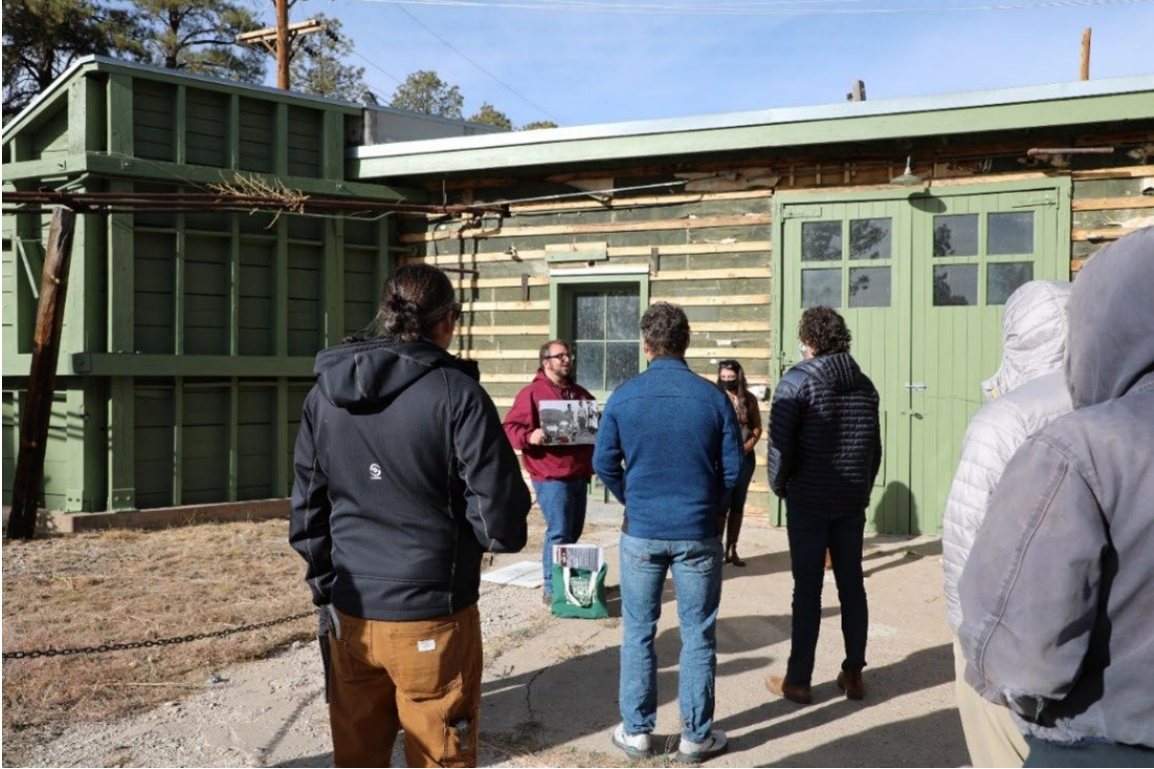
Figure 3-1. LANL tour at V-Site. Note that asbestos siding shingles have been removed and prepared for replacement of replica non-asbestos siding shingles.
