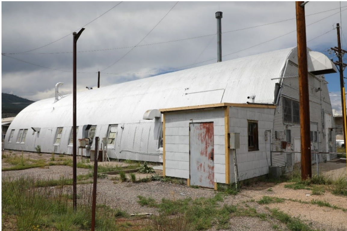
Figure 3-2. Oblique view of Technical Area 22, Building 1 Quonset Hut.
