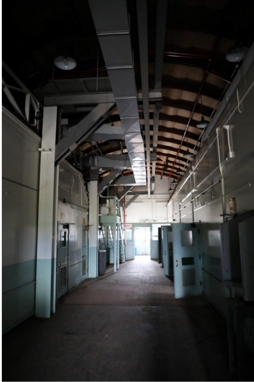
Figure 3-3. Interior view of Technical Area 22, Building 1 Quonset Hut.
