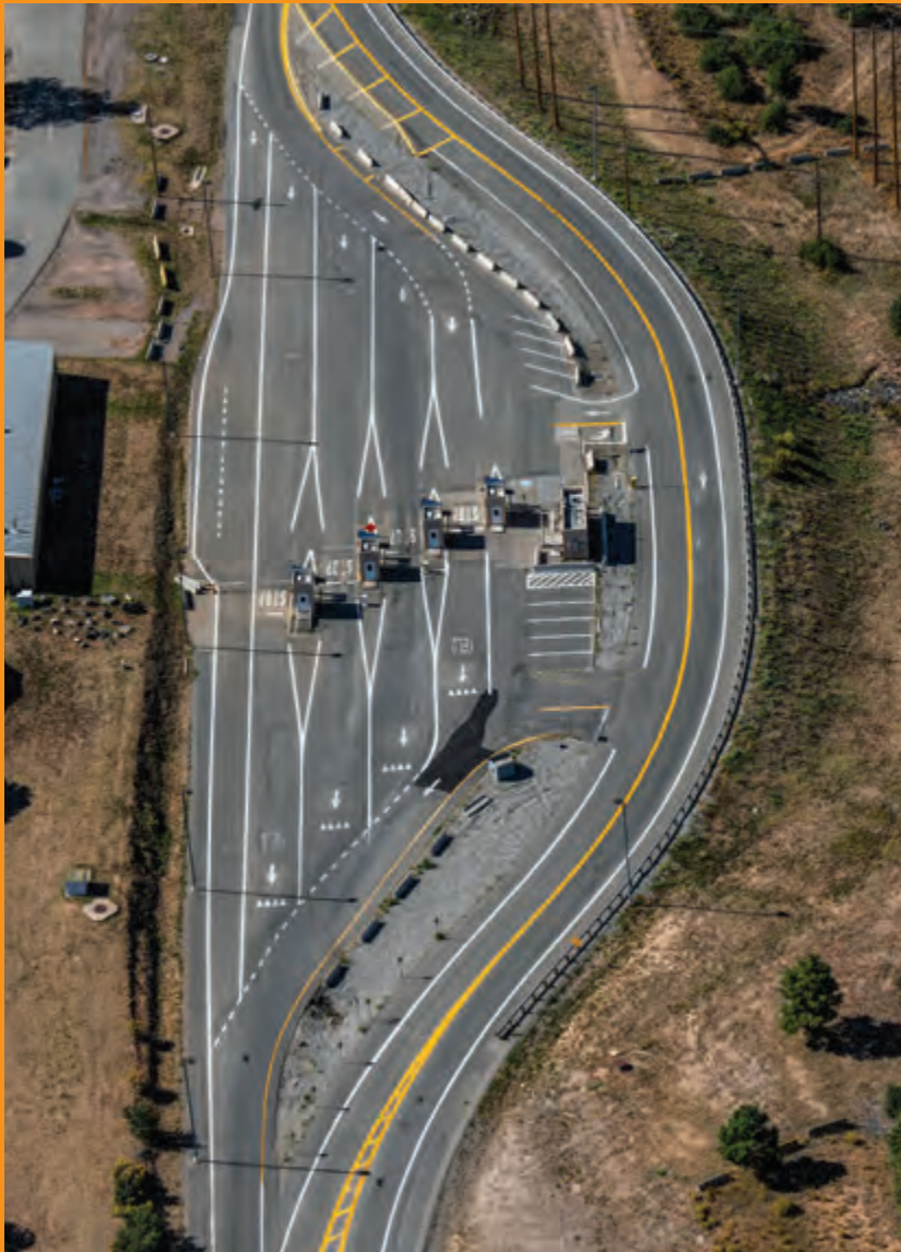
Aerial view of a vehicle access portal along Pajarito Road.
