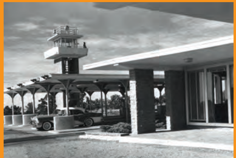
East Gate Security Station.
