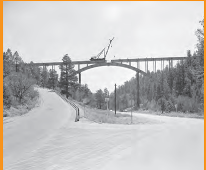
Construction of Omega Bridge over Los Alamos Canyon, 1951.
