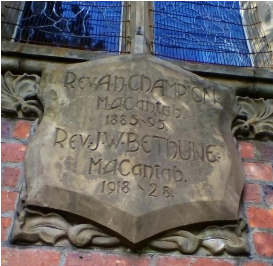
One of the major features of the exterior walls are shields bearing the names of past headmasters from the foundation of the school in 1846.
