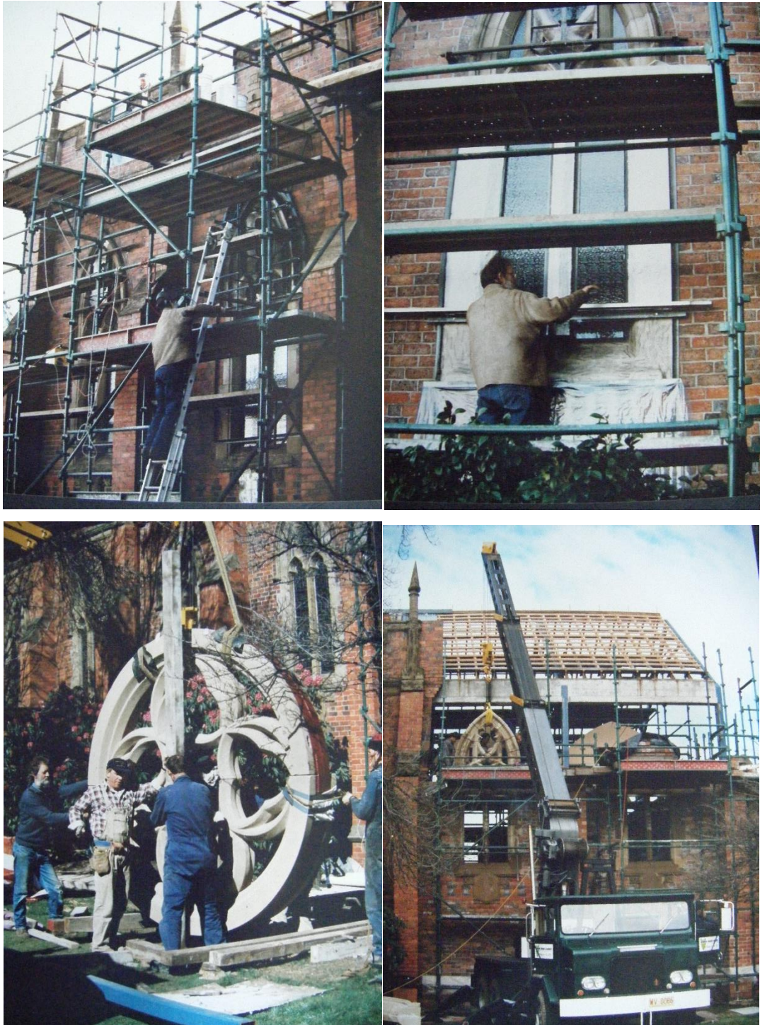
Composite during construction
