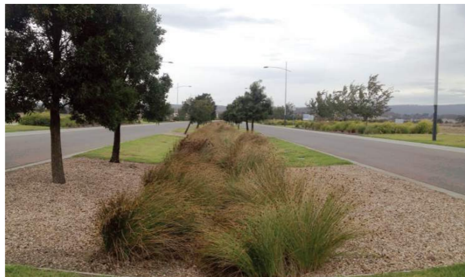
Entry drive with swale
