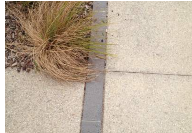
Exposed concrete aggregate pavement + contrast brick pavers
