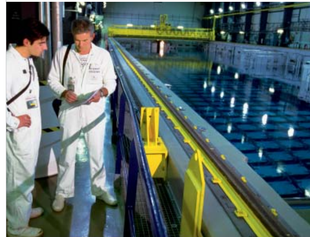
Fuel discharged from nuclear power reactors is shipped to the La Hague plant, where it is cooled in storage pools.
