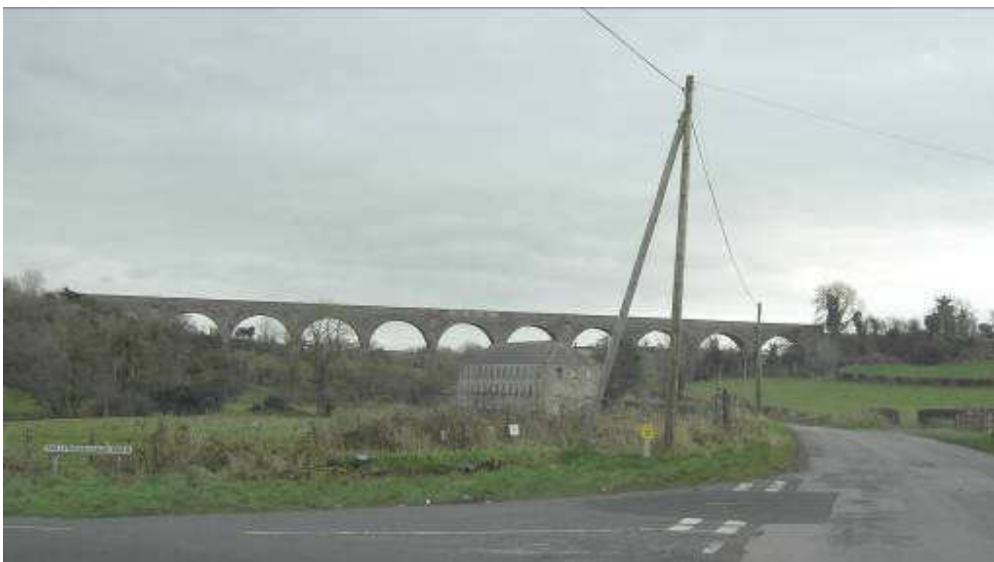
Plate 96: Tassagh Railway Viaduct, Armagh (No. 108)
