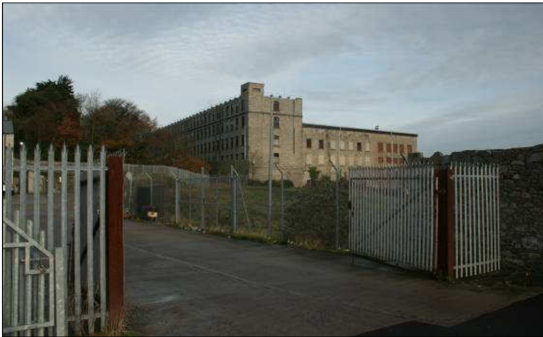
Plate 78: Bessbrook former mill, Co. Armagh (No. 36)
