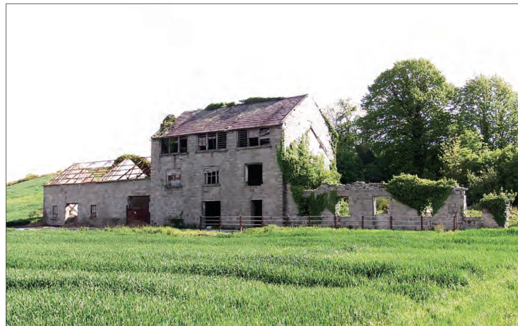
The upstanding remains of the bleech mill at Carnmeen (Site 24)
