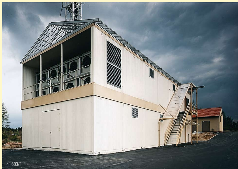
FIG 2 Lightweight two-story transmitter building.
