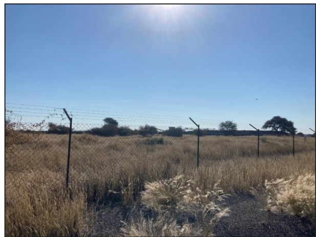
Figure 7: View of the Wessels Mine perimeter fence
