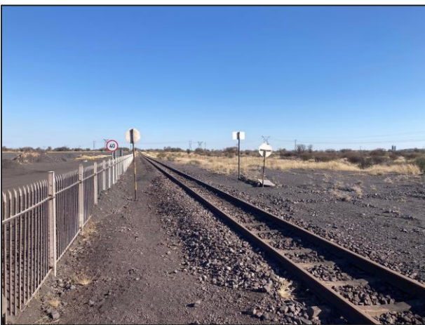
Figure 6: View of the existing railway line
