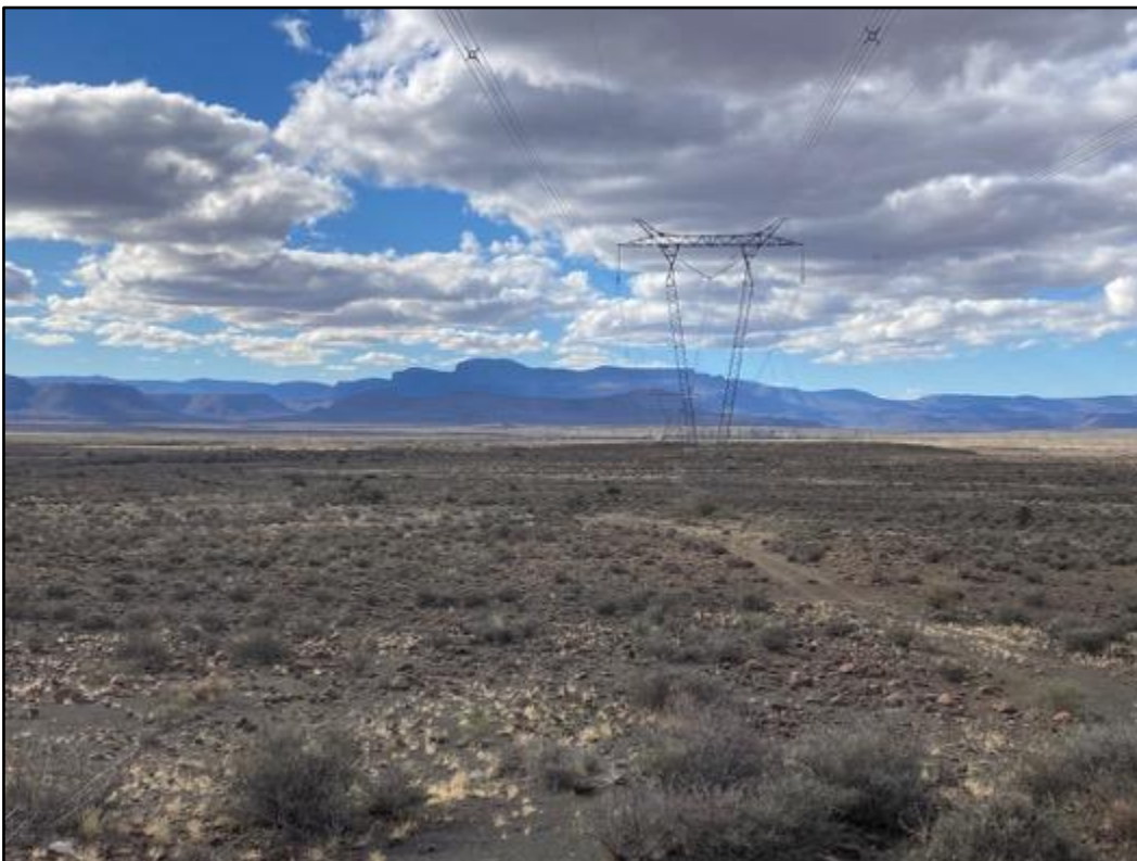
Figure 17: View along existing power line towards Dröerivier MTS.
