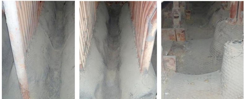
Original ISOMEMBRANE® Installation in 1994, photos taken May 2013
