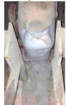
ISOMEMBRANE® in the 4 th & 5 th stages of installation
