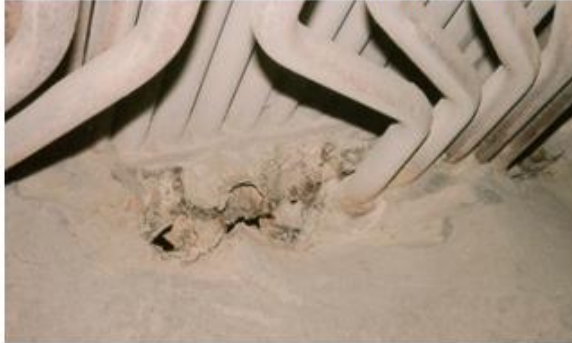
Prior to installation of ISOMEMBRANE® in 1994
