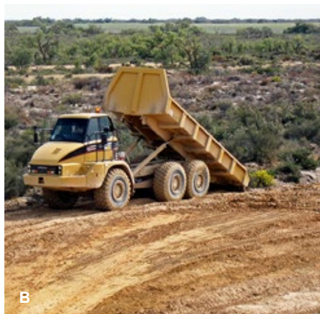
Construction of the vegetation direct transfer (VDT) trial at Eneabba, Western Australia. Excavator cut (A) and direct placement (B) of ~30 cm soil with largely intact kwongan vegetation. Photos: C. Payne.
