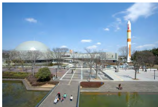
Fig. 1 – External View of Tsukuba Expo Center (planetarium dome visible on left side)
