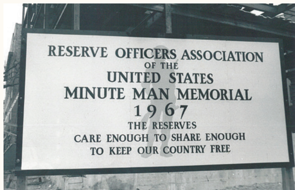
The world learns about the new Minute Man Building.
