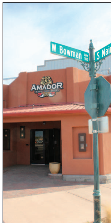
The front entrance
