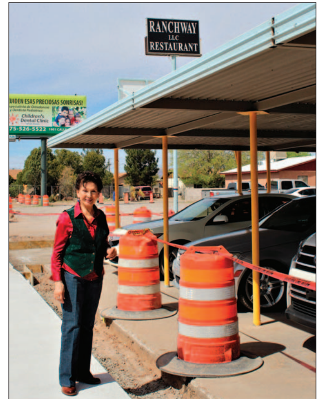
Owner Elsa Rodriguez poses outside Ranchway Restaurant, next to the orange construction barrels on Valley Drive.
