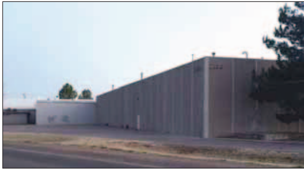
The former Coca Cola bottling plant at 2100 S. Valley Drive is now Las Cruces Studios.
