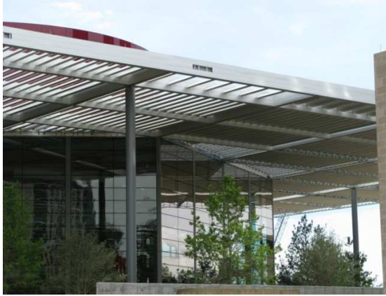
Winspear Opera House Sun Shading en Dallas
