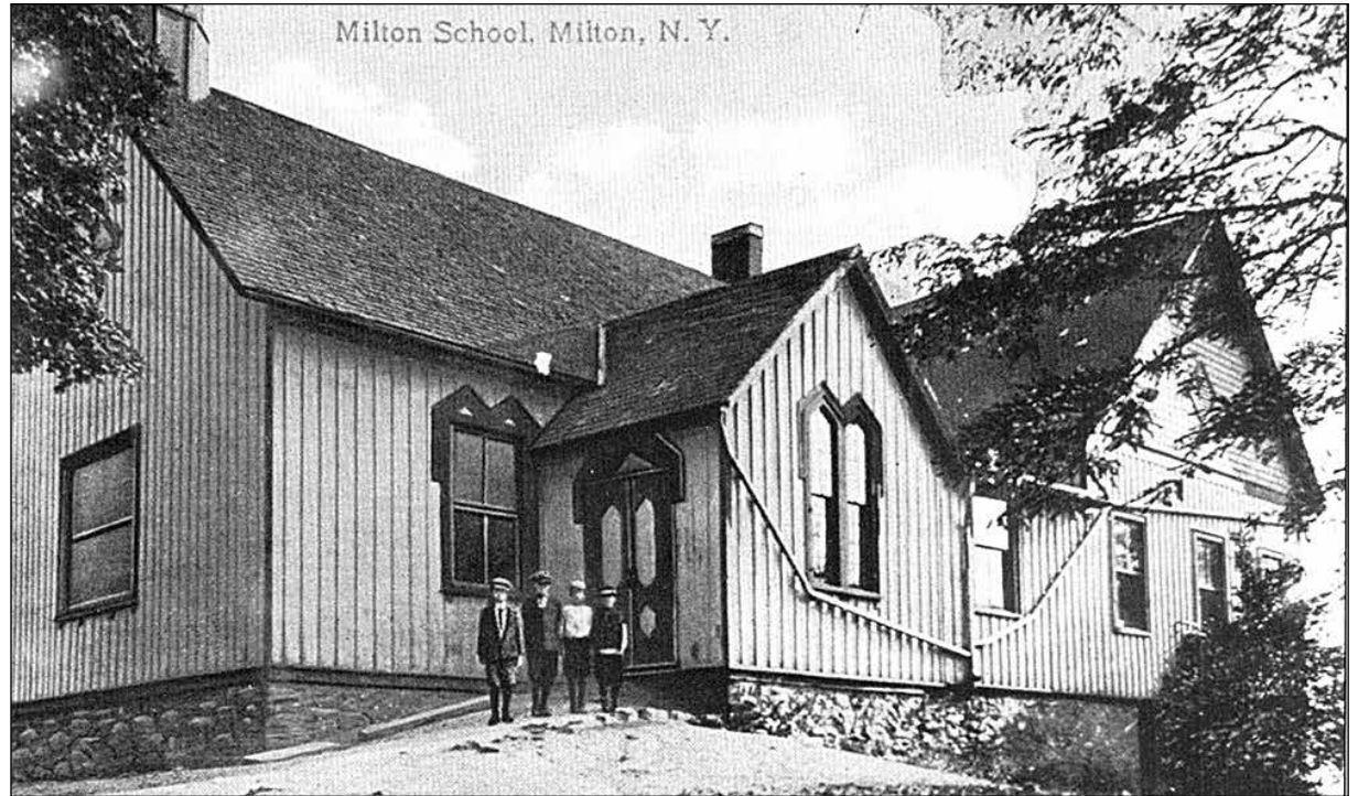
Sands Avenue School, Milton. The center room was the original one-room school built in 1840. The school had a small hall for the boys and one for the girls with about 150 desks. A long platform ran the length of the school for reciting and a large wood stove kept everyone warm.
