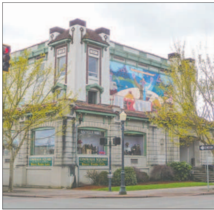
ON PEARL STREET in Centralia sits Centralia Square, home to 80 antique dealers in one and a half stories. The mall was originally a regional Elks lodge and the top floors are currently being refurbished.
