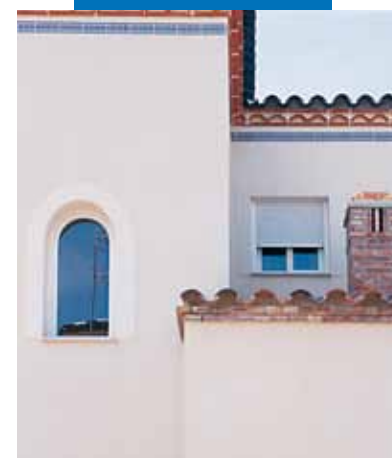
End result after application process of Mapefront Raspat
