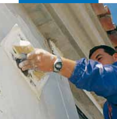
Trowelling Mapefront Raspat
