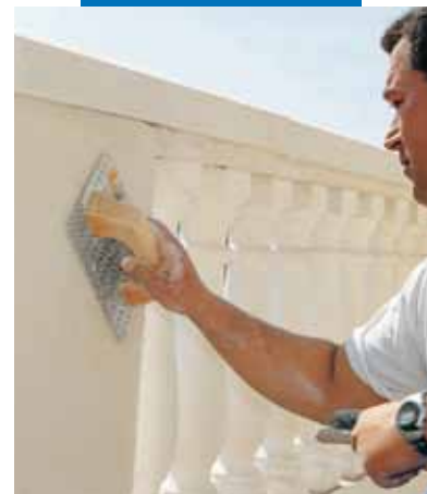
Scraping Mapefront Raspat
