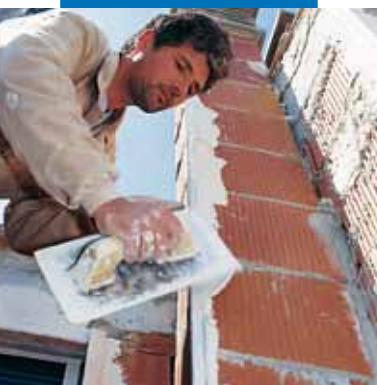
Controlling surface levelling with rails
