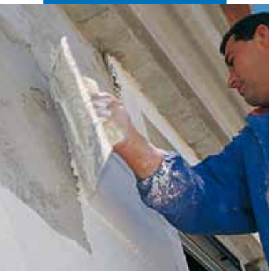
Application of Mapefront Raspat
