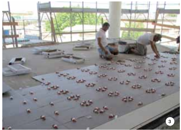
In the interiors, after building the screeds with TOPCEM PRONTO, the porcelain tiles were installed with KERAFLEX MAXI S1 cementitious adhesives. Joints were grouted with ULTRACOLOR PLUS high performance mortar, both in interiors and exteriors.
