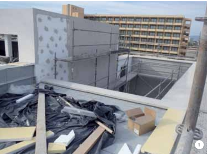
PHOTO 1. The MAPETHERM TILE SYSTEM was used for external thermal insulation.
