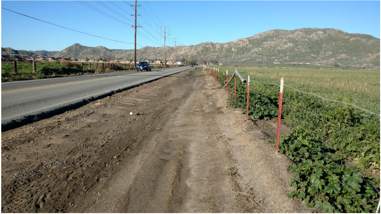
Photograph 5 – Ditch north of Esplanade Avenue and west of Cawston Avenue, facing west. Agricultural lands to the north (right).
