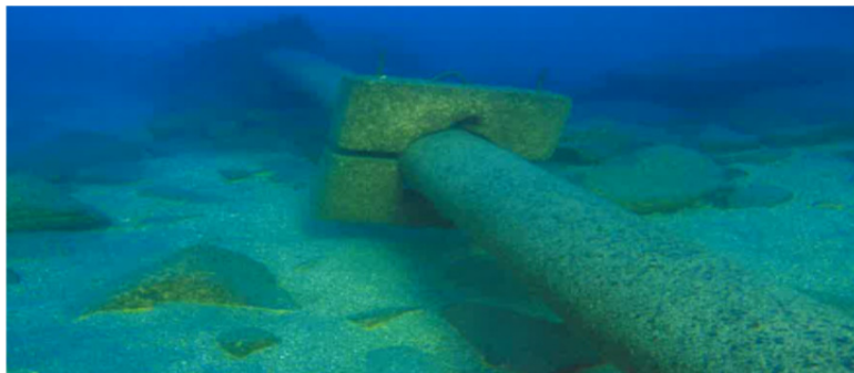
Photo 3-1 Pipeline and Anchor Block
