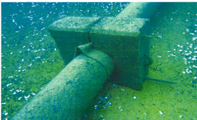
Photo 3-1. Pipeline & Anchor Block
