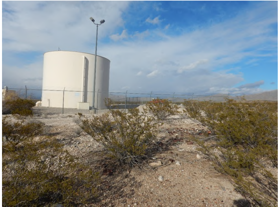
Photograph 1: Overview of Project from Southwest corner, facing northeast.
