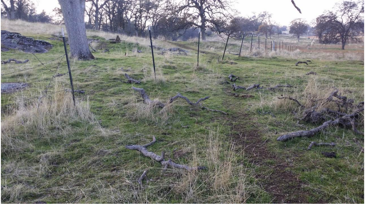
Broken fencing still in disrepair at the south edge of northeastern arm of open space preserve. Cattle trail from neighboring property (background) can enter open space preserve (foreground).
