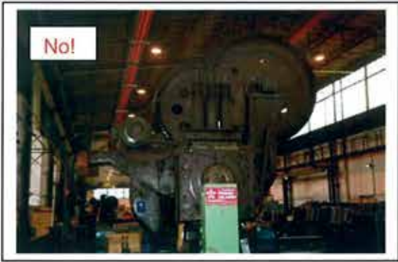
Figure 4.8a: Unprotected belt and wheels – beyond 2,5 m height it is dangerous for employees in direct way, but above 2,5 m e.g. the chain or hook of crane can be caught and a catastrophe initiated...
