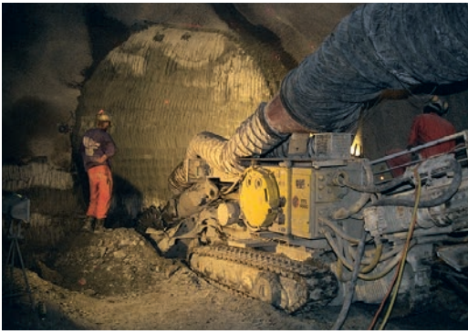
9. Construction on the LHC transfer tunnel.
