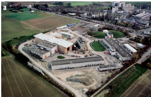
29. Two aerial views of the major surface construction sites; (a) the ATLAS site at Point 1; and (b) the CMS site at Point 5.
