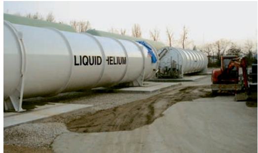
59. 120 m 3 vacuum-insulated storage reservoirs for liquid helium.
