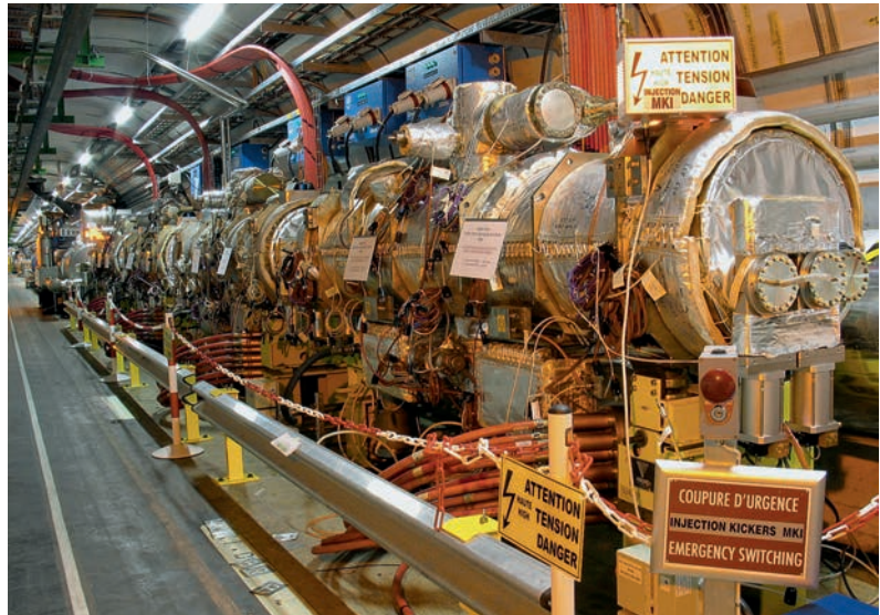
70. Sequence of four injection kickers at Point 8 (photo V. Mertens).
