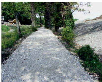
31. Landscaping with the disposed spoil of the LHC construction sites, used to reinforce a centuries-old Roman path in the vicinity of Cessy.
