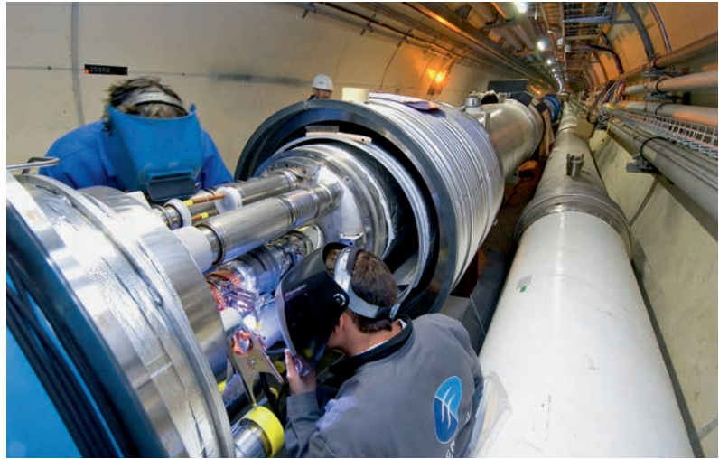
47. View of LHC in tunnel, showing string of magnets and cryogenic distribution line.
