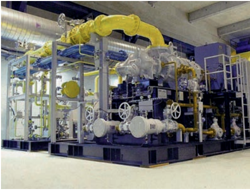
54. 1.8 K refrigeration unit for LHC: (top) room-temperature compressors, (bottom) cold box with cryogenic compressors.
