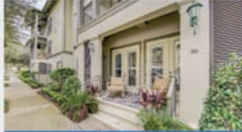
601 SYCAMORE ST You can't get closer to downtown Celebration than this newly renovated Carlyle smart 2/2 condo with attached garage - $355,000
