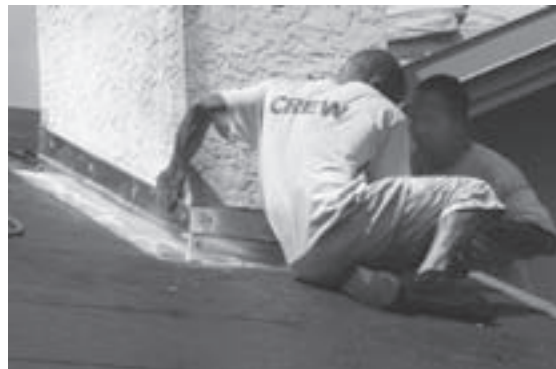
Repairs. We are the Roof Repair Experts!
