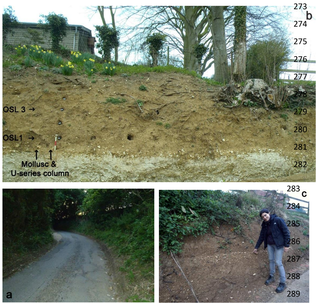
290 Figure 3. (a) Woodland Road, Lyminge hollow way west of sampled section; (b) sampled lynchet 291 section showing position of OSL and mollusc samples, scale 30cm; (c) the Phase 1 lynchet to the right 292 of (b) (photos M. Bell).
