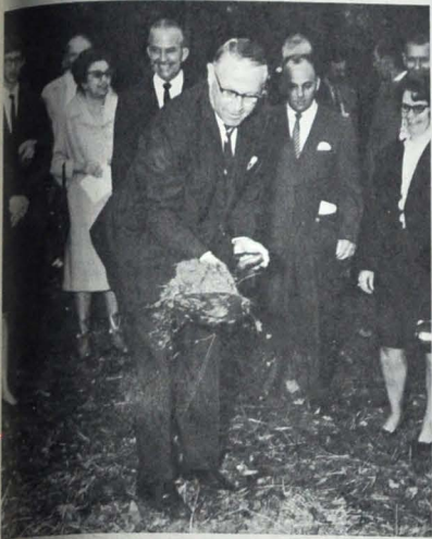
GROUND-BREAKER—Scooping up a shovelful of dirt at the site of the new Central High School is Principal W. Hobart Millsaps.
