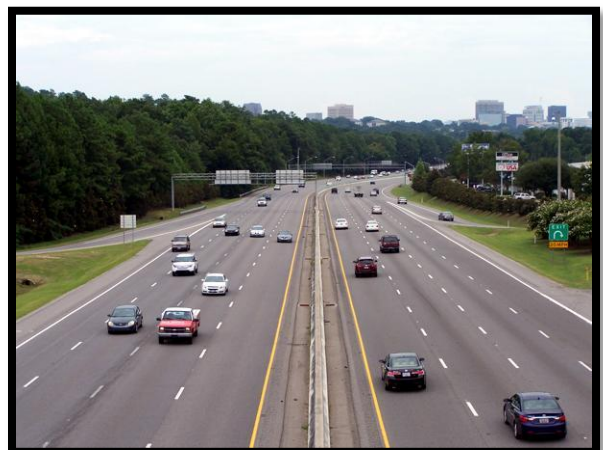
I-126 near Greystone Boulevard
