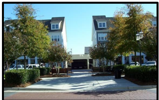
Birkdale Structured Parking, Huntersville, NC
