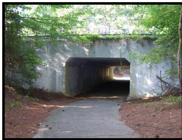
Harbison Pathway Tunnel under Broad River Road
