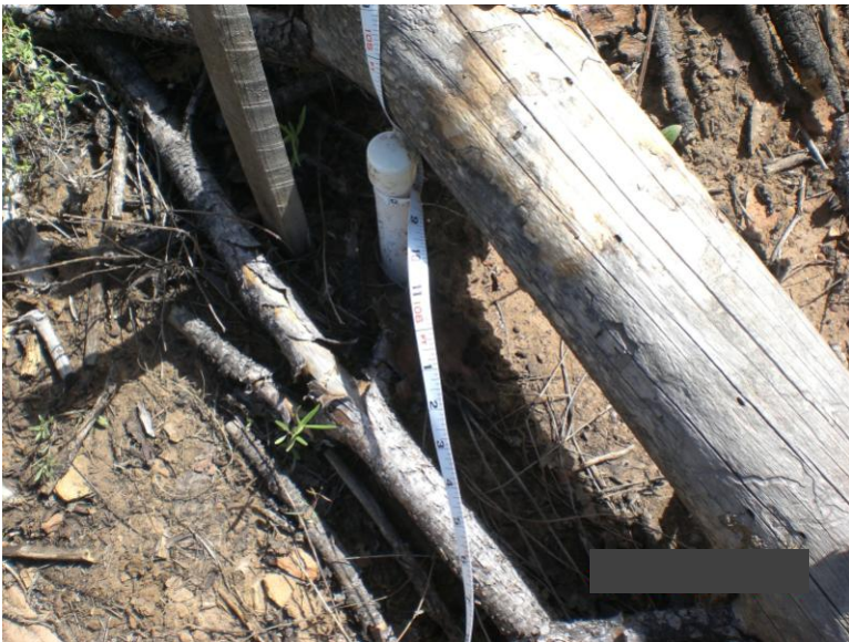
Figure 8. Old rebar hidden beneath log
