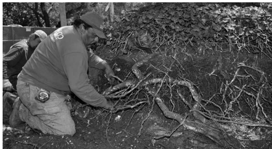
Top: Pamela Seager with contractors in Barnyard, 2011. Photo by Cristina Klenz. Middle: At the 2009 opening of the Native Garden, Pamela Seager and Bart O'Brien, director of horticulture at the Rancho Santa Ana Botanic Garden. Bottom: Contractors hand-excavating tree roots in barnyard, 2010. Photo by Cristina Klenz.
