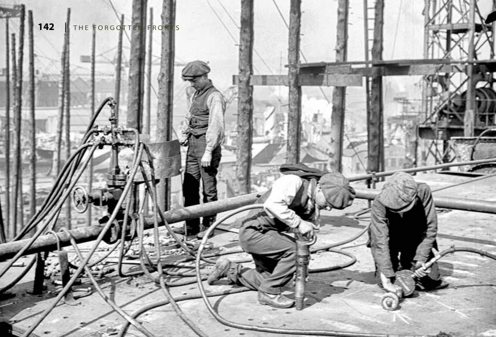
12.7 Worker operating pneumatic hammer on a merchant ship during construction © IWM
