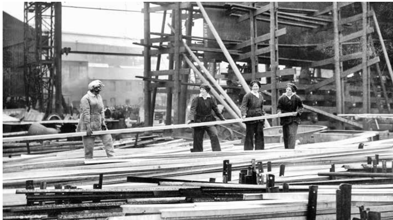
12.9 Female ship yard workers preparing shoring timbers at a naval ship building yard © IWM
