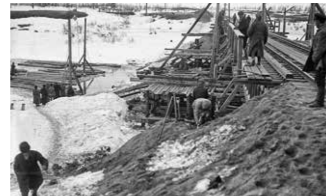
16.10 Constructing a railway bridge in Shuyenetskaya © IWM
