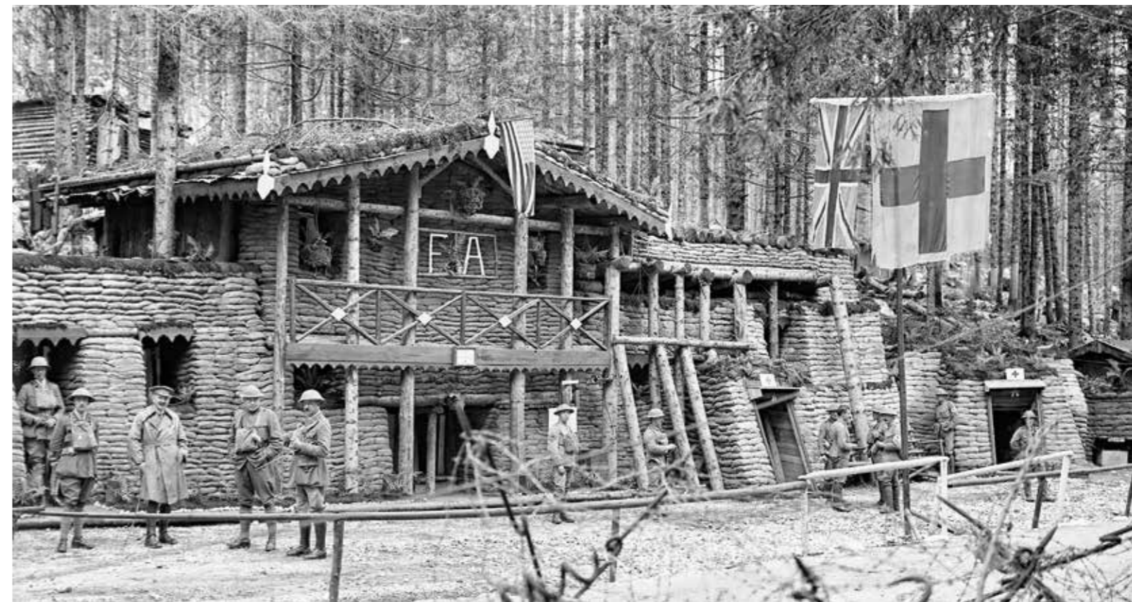
6.5 Soldiers of the Royal Army Service Corps outside a Field Ambulance Station. Note extensive use of sand bags for building protection © IWM
