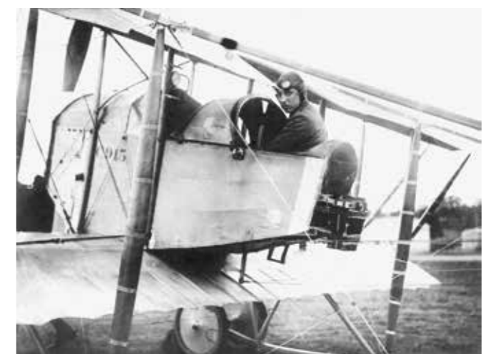
10.5 A Type aerial camera fixed to a vertical mount aft of the cockpit of a Caudron G.3 C945 of the Royal Flying Corps, 1915 © IWM
