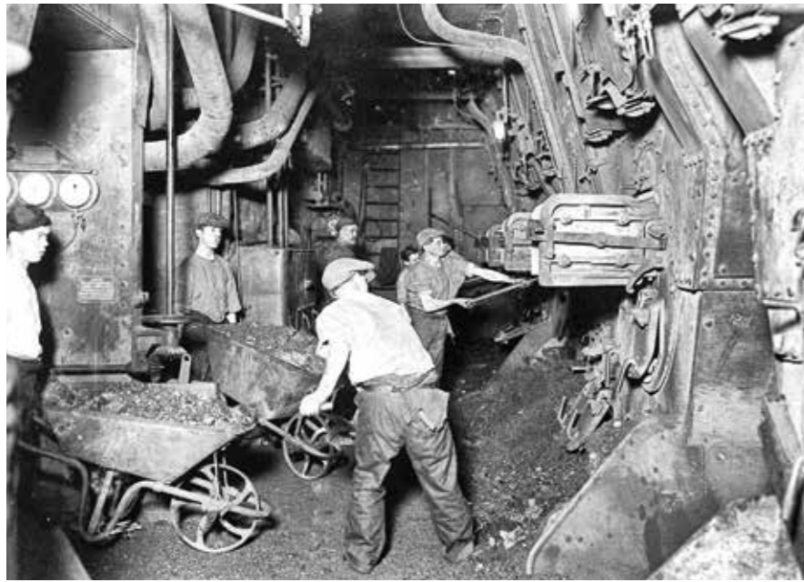
12.4 Men working in the stoke hold of a merchant ship © IWM
