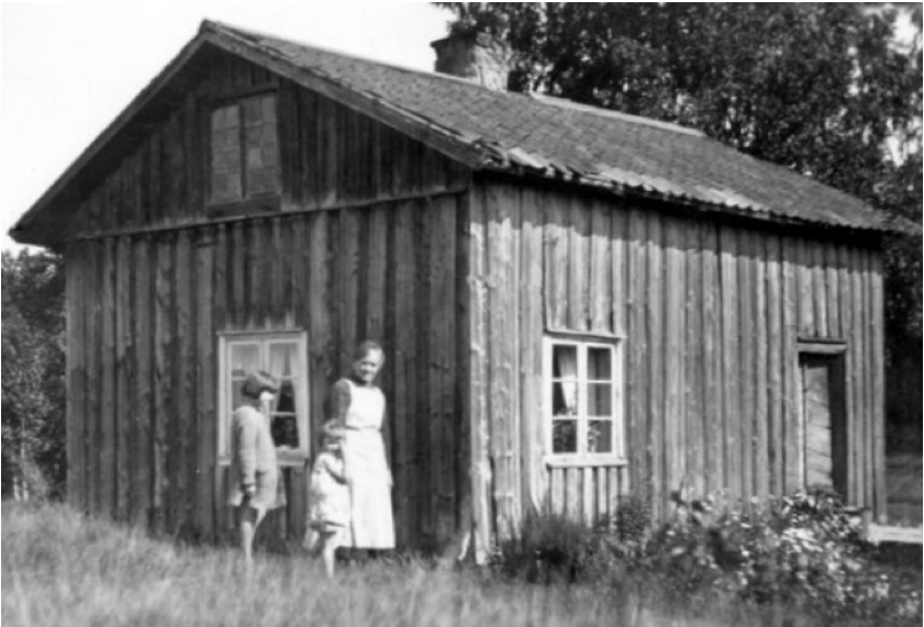
Anders' mother (Gunvor Thorstenson Rhodin) and aunt (Ingrid Thorstenson Froste) as children at a neighbor's home ( torp ) in södra Slotteviken, right across Lake Råvarpen from Branterud, ca. 1928. This one-and-a-half story timber house ( enkelstuga ) with offset front door and large hearth and chimneystack would have been almost identical in layout to the Färdig–Gustafsson house, built at about the same time in the mid-1800s. Photo by Gunnar Thorstenson, Anders' grandfather.
