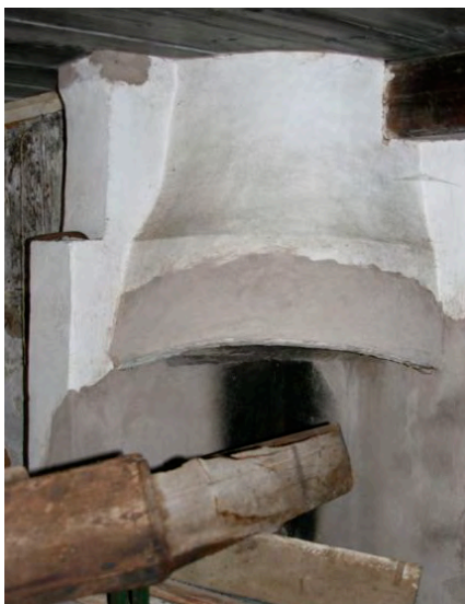
The traditional heating for homes in the area was an open hearth with gypsium cupola in the main room. This one is from the old house at Slotteviken (see photo on p. 24) and is being restored. Photo by Anders Rhodin.
