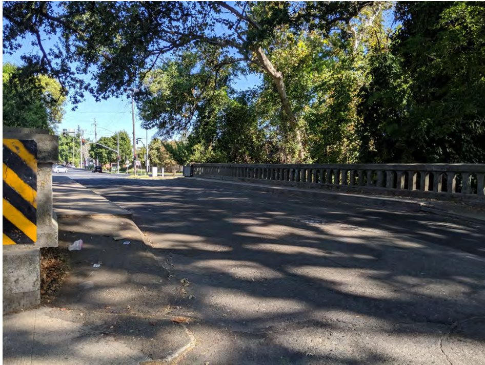
Salem Street Bridge Looking North
