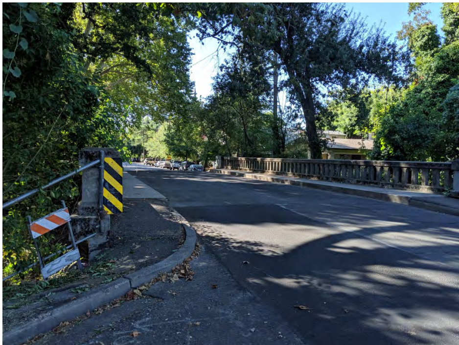
Salem Street Bridge Looking South
