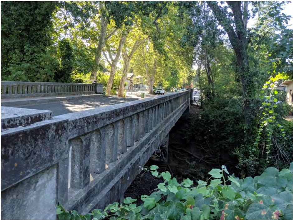
Salem Street Bridge Looking South
