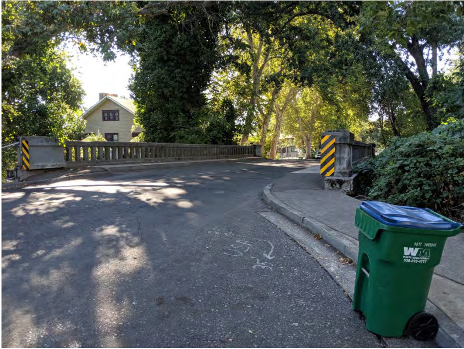
Salem Street Bridge Looking South
