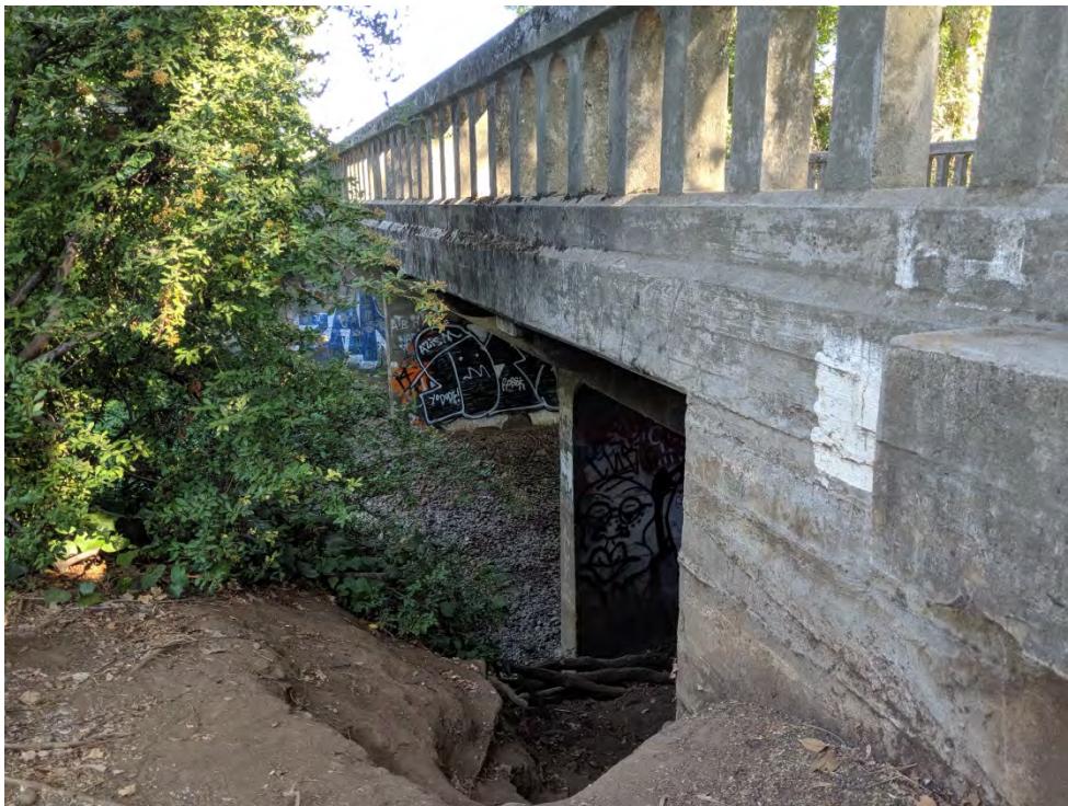
Salem Street Bridge Looking North
