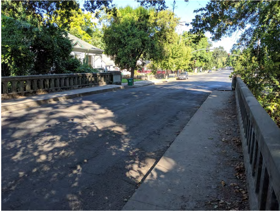
Salem Street Bridge Looking North
