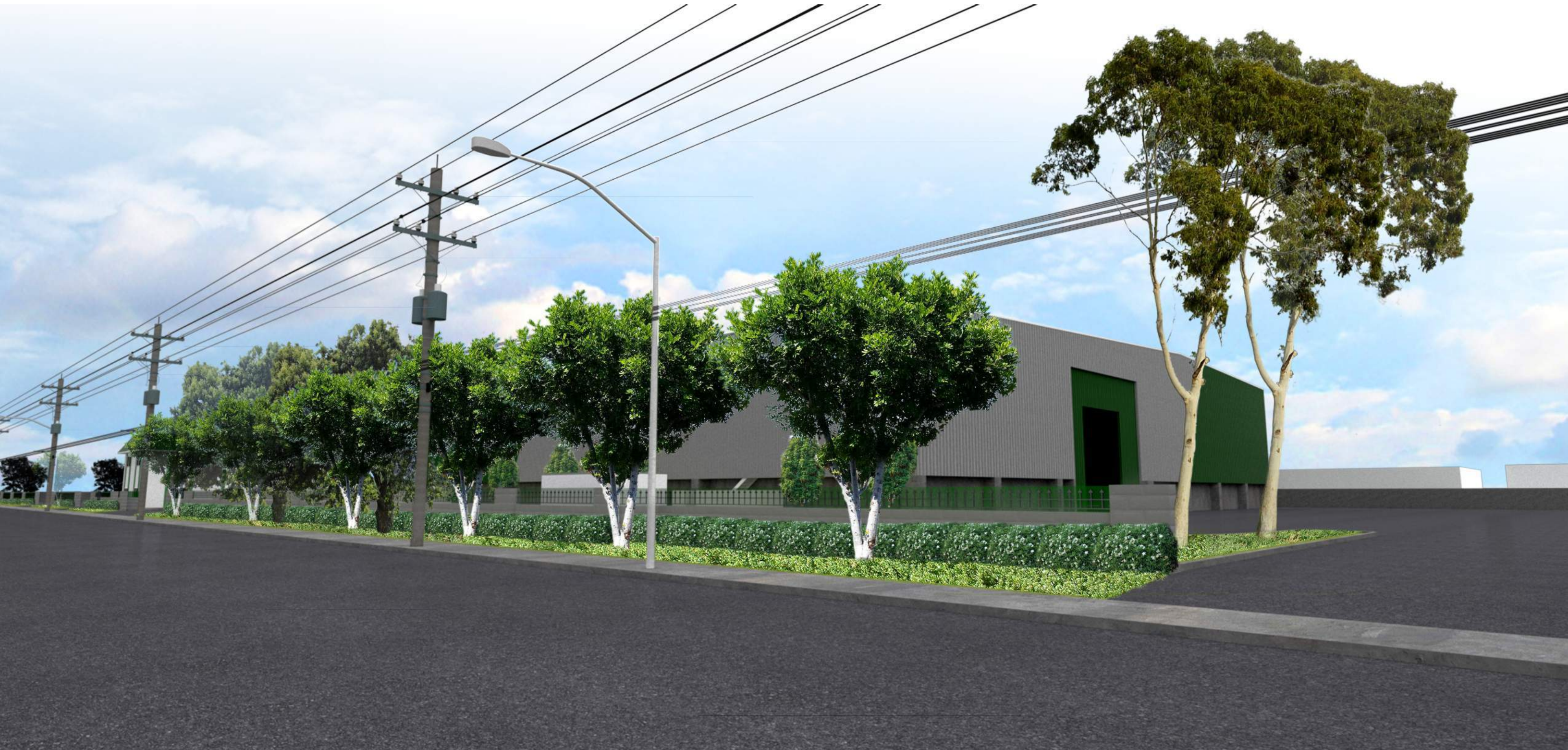
VIEW ALONG WEST FRANCISCO STREET LOOKING NORTHWEST AT EXISTING TRANSFER STATION
