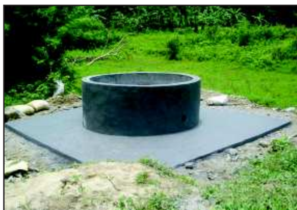
Plate 2. Well constructed by WUA
