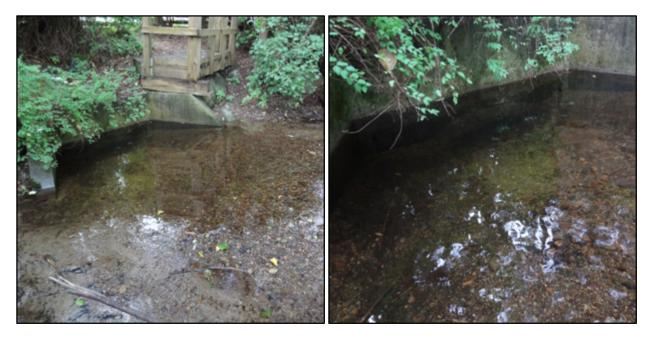
**Figure 19**: A pre-cast concrete headwall was installed at Spanish Bank Creek. The pre-cast concrete headwall is located at the north end of the wood stave culvert that spans under NW Marine Drive (left). Accretion of sediment has filled in the lower reaches of Spanish Bank Creek, thereby impeding flow through the wood stave culvert (right; Reynolds, 2016).
