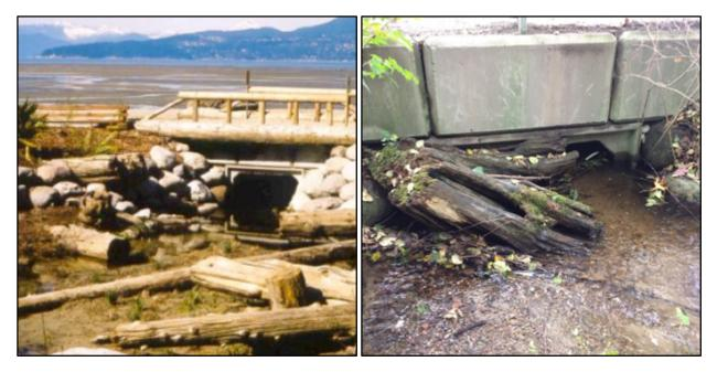
**Figure 18**: The lower reaches of Spanish Bank Creek have been filled with sediment. Installed in 2000, the concrete box culvert pictured above is 6 m long, 1.2 m tall, and 1.8 m wide (left; Hollick-Kenyon, 2002). After 16 years only a fraction of the culvert is passable due to build-up of sediments (right; Reynolds, 2016).
