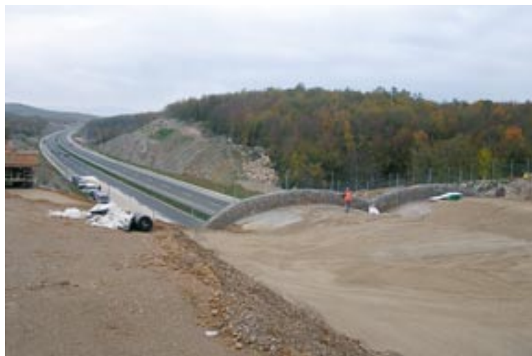
Figure 100. The Medina gora green bridge on the Zagreb – Split motorway, the Otočac – Lički Osik section (J. Kusak)
