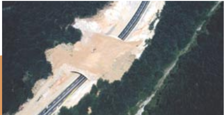
Figure 28. Green bridge “Dedin” on the Zagreb-Rijeka highway, the first green bridge for animal crossing in Croatia (F. Knauer)
