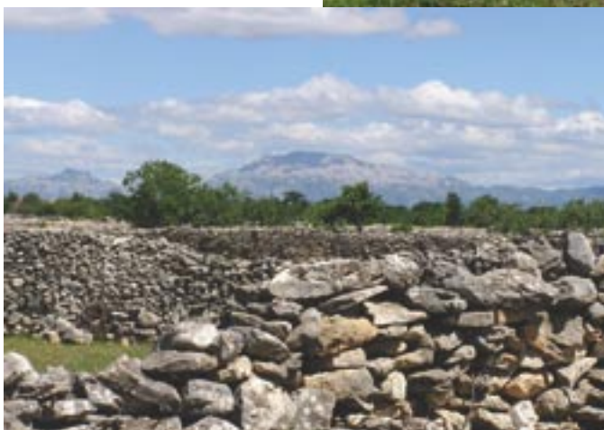
Figure 71. A drystone wall in Dalmatia (P. Štrbenac)
