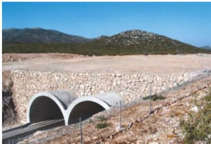
Figure 40. The Osmanovac green bridge on the Zagreb-Split motorway - Prgomet-Dugopolje section, constructed due to the presence of wolves (J. Kusak)
