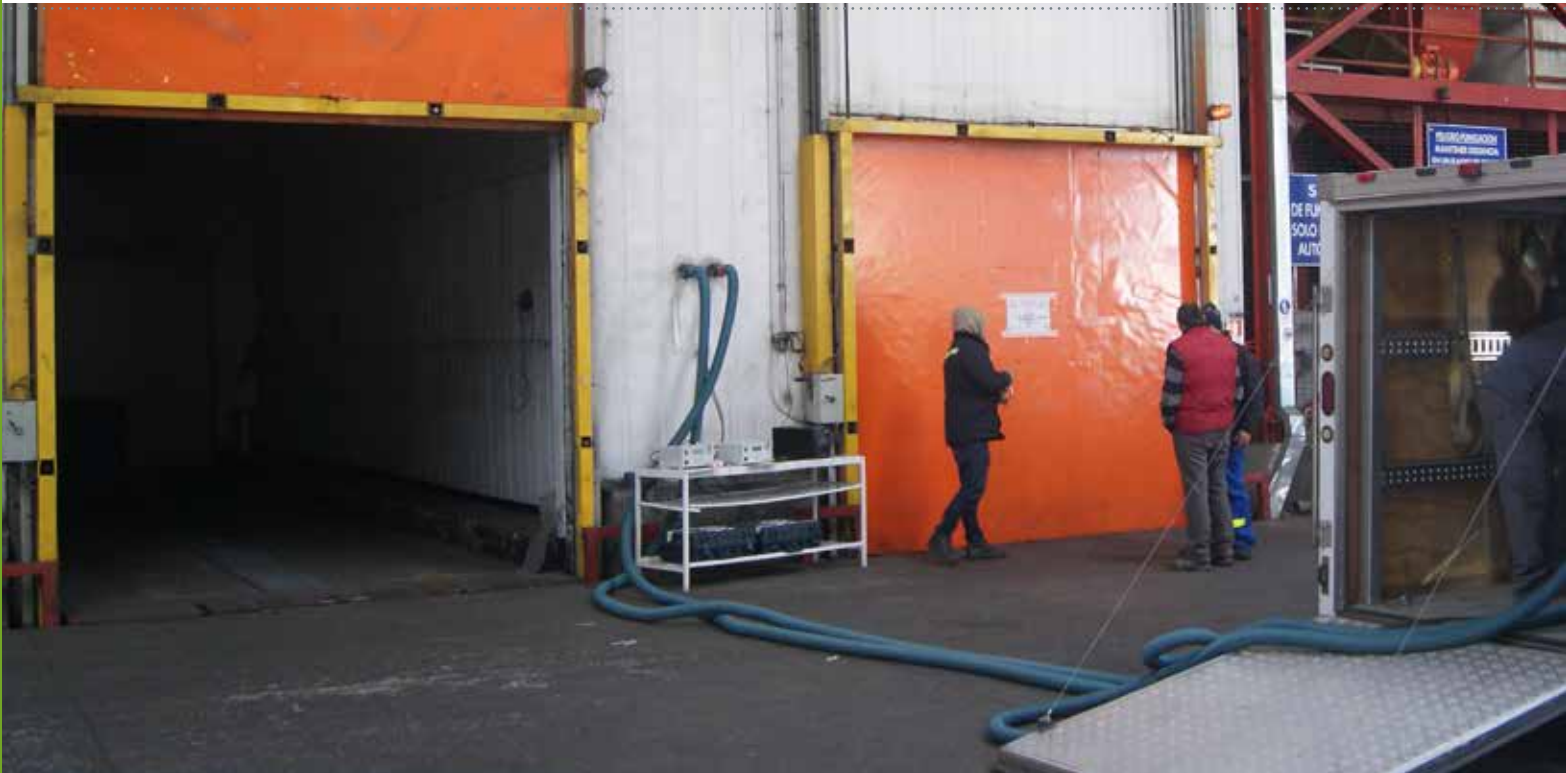
Large controlled atmosphere rooms open (left) and closed (right) for cold storage phosphine fumigations.
