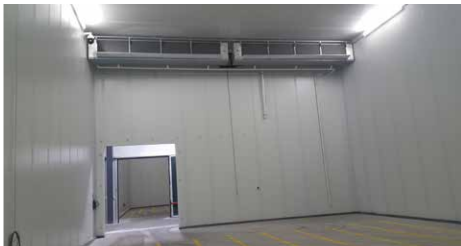
Figure 1. Due to treatment durations that are long, relative to those for methyl bromide, cold-storage phosphine fumigations can be conducted in large controlled-atmosphere rooms, maintained under cold-storage conditions, as a means to minimize disruptions to export throughput.
